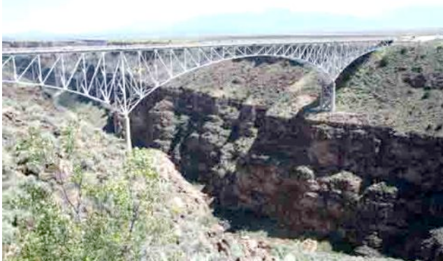
Bridge over the Rio Grande - near Taos.
